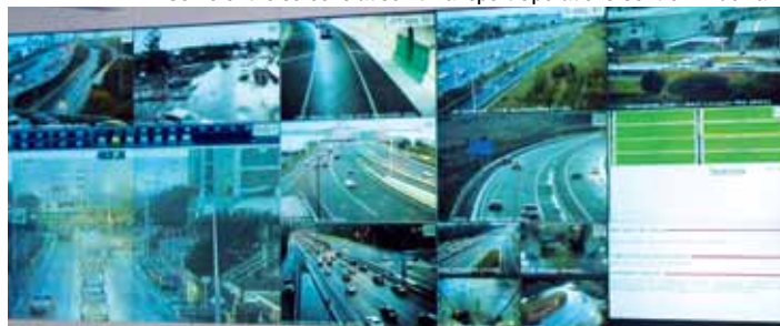
Some of the screens at Joint Transport Operations Centre in Auckland
